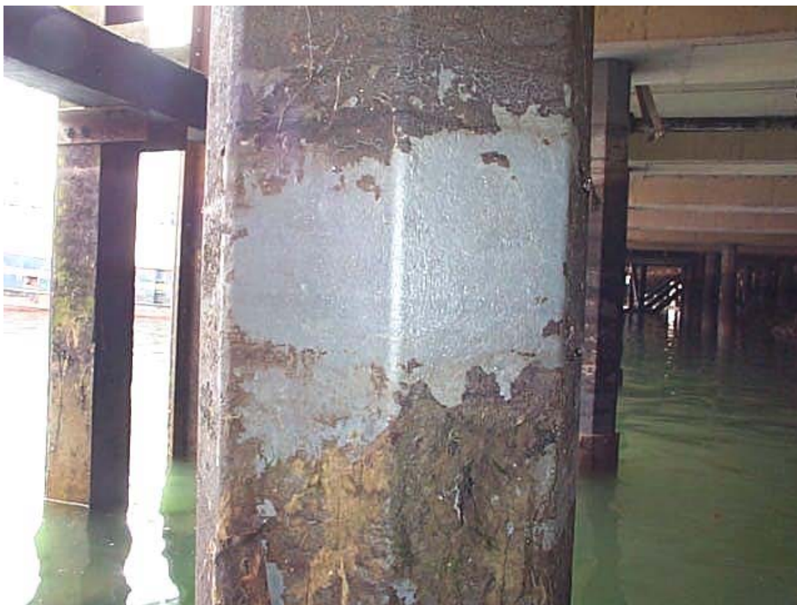
Plate 1. Area of pile cleaned for inspection
