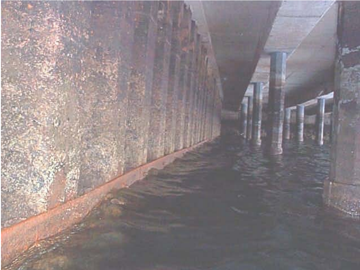
Plate 4. Steel plates to Wave Curtain.
